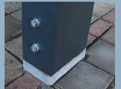
Visible connection support/screw foundation (flange plate screw head and support above roadway surface)
