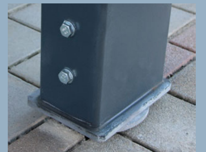
Visible connection support/screw foundation (flange plate screw head and support above roadway surface)
