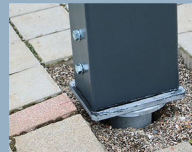
Visible connection support/screw foundation (flange plate screw head and support above roadway surface)
